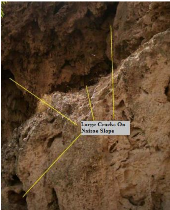
Fig. 4. Development of new cracks and voids after a seismic episode
