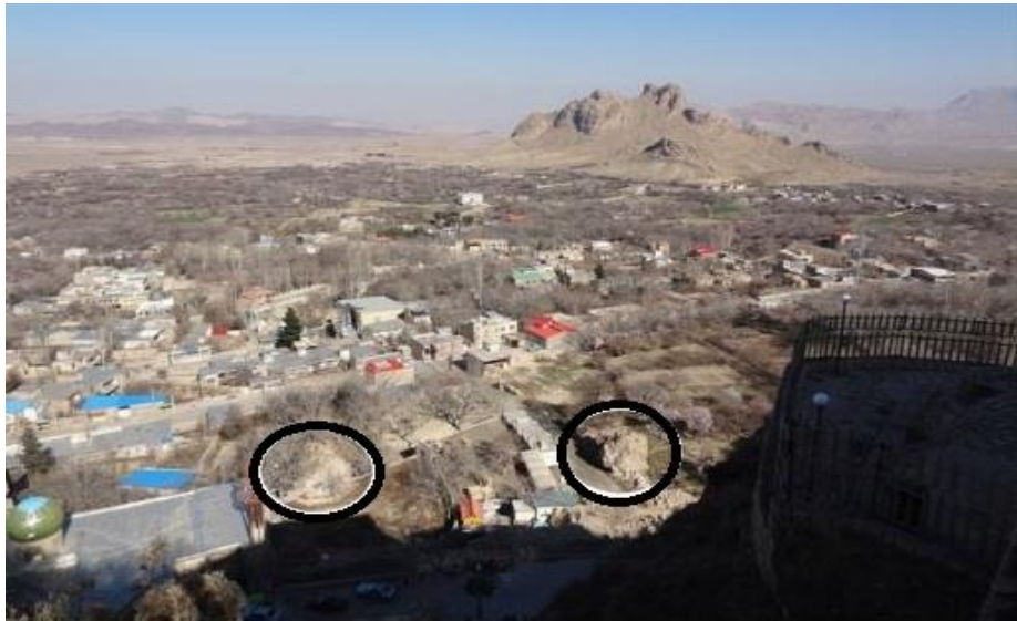
Fig. 3. Approximately 30 years ago, an earthquake caused these two massive stones to separate from the wall and fall into the inhabited area below.
