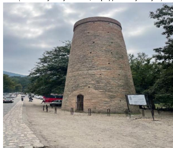
Fig. 4: Water pressure relief tower, By Authors
