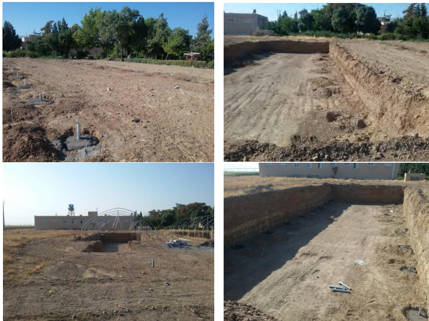
Figure 2. Different stages of greenhouse construction
