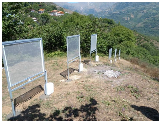
Fig. 6. A view of the systems installed in Vishki village
